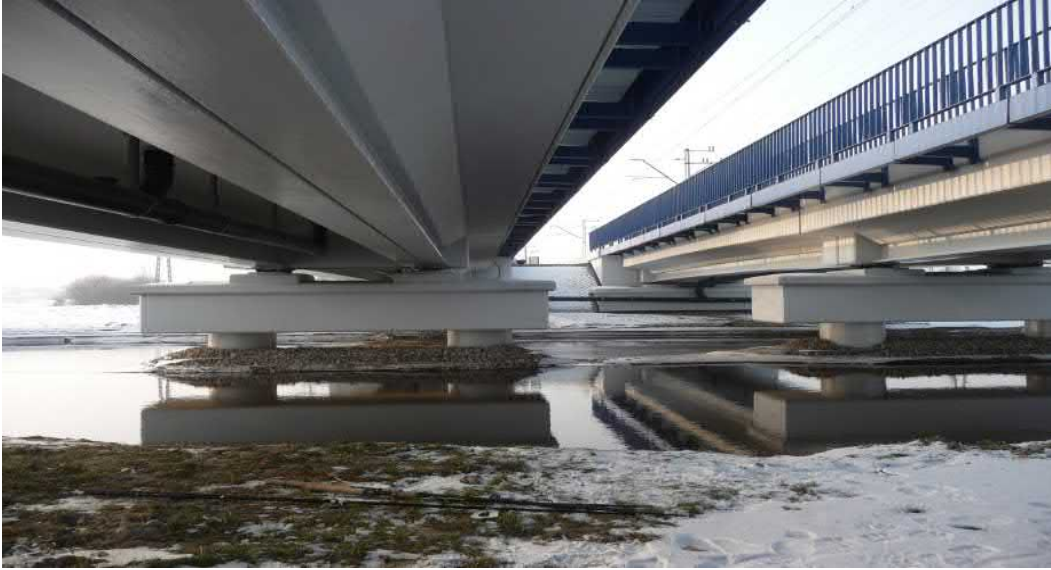
Figure 36: Bottom view of “Wiarna Rzeka” bridge.
