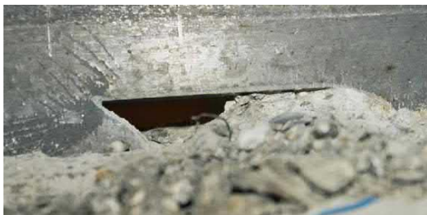
Figure 19: Plastic deformations of steel dowels in the region of the sharp notch in the SA shape (push-out specimen [30]).
