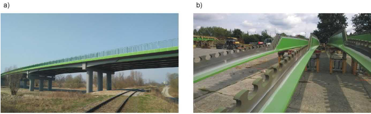
Figure 1: Steel–concrete hybrid beams of innovative composite bridge constructed using composite dowels in Poland, 2016.
