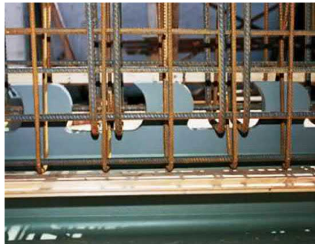
Figure 11: Modified SA shape (without the sharp notch) used in the Vigaun Bridge [7].
